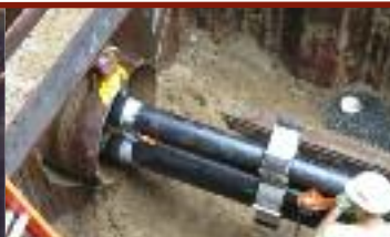
Ronkonkoma Hub Pump Station
