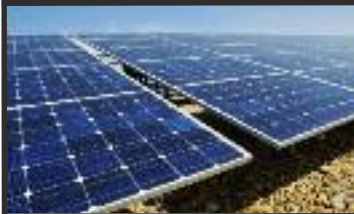
Smithtown Solar Photovoltaics
