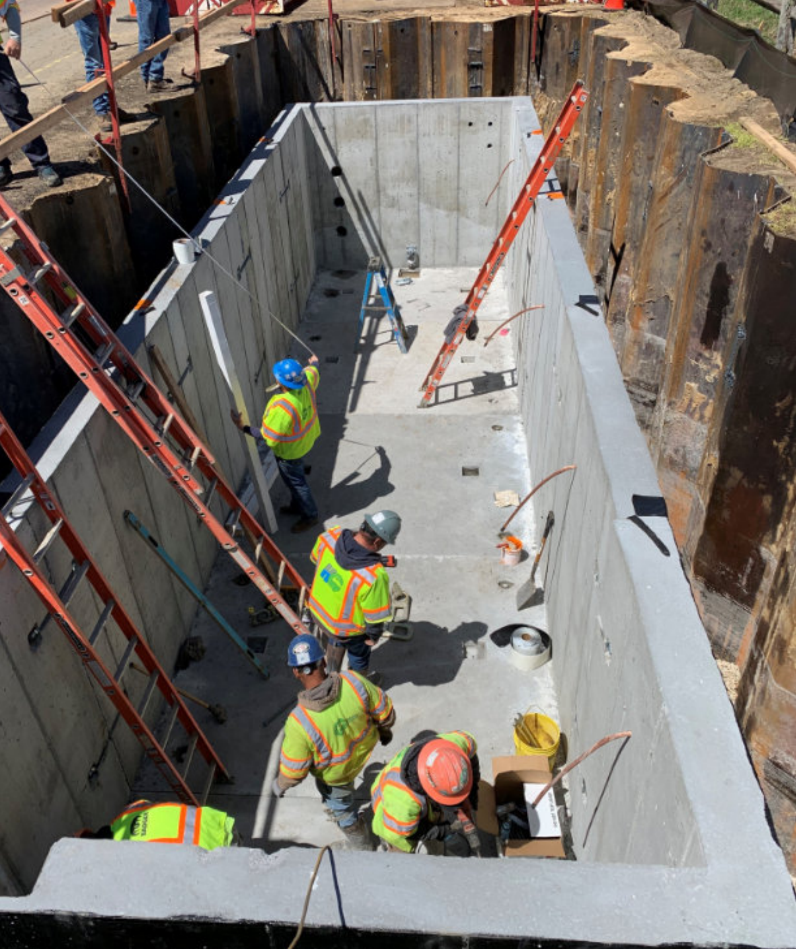
TRANSITION JOINT BAY (TJB) INSTALLATION BEACH LANE
