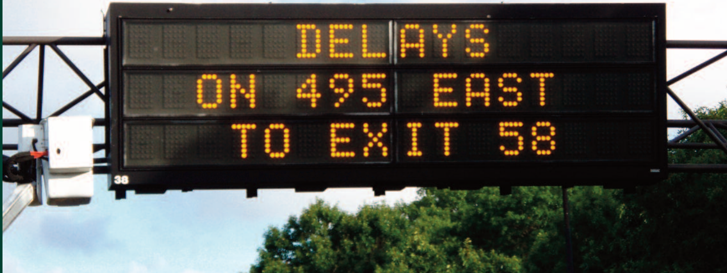
Overhead signs inform motorists of conditions ahead
